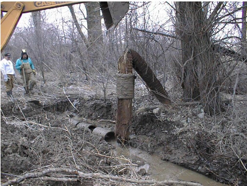
Figure 4. The same 15 inch tile as in figure 3. Tree roots entered through the gaps between each tile. The roots are often fine and fibrous and packed very tight within the drain.
